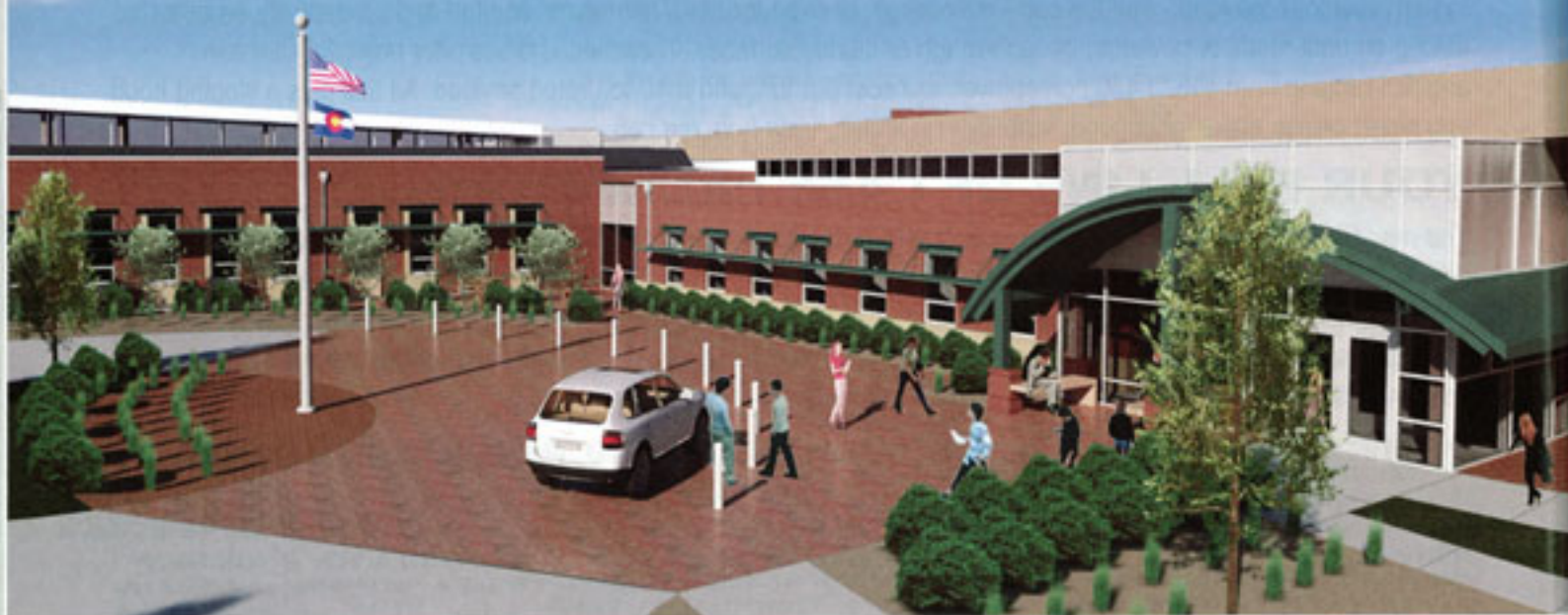
» Loveland, Colo.-based Alliance Construction is underway on a new project at Morgan Community College.
